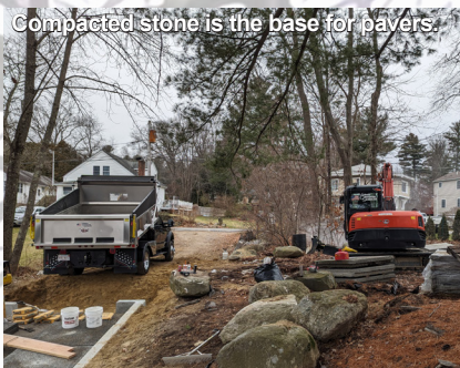
Fine gravel for the base is delivered.
