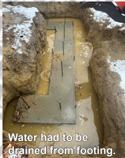
This concrete footing cannot be seen under the finished installation of pavers.
