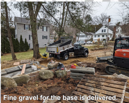
Compacted stone is the base for pavers.
