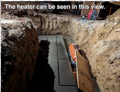
Water had to be drained from footing.
